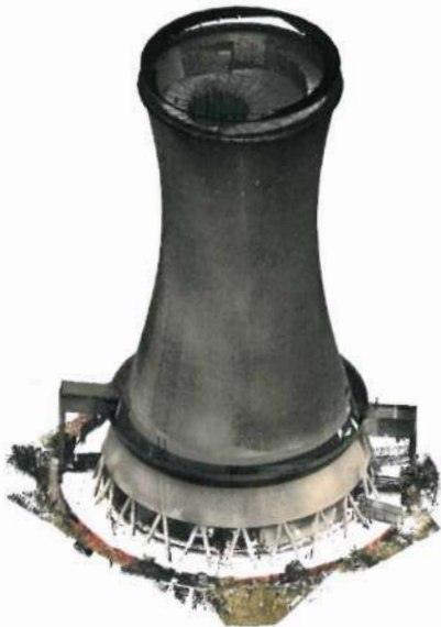
Fig. 2. Point cloud of the hyperboloid hyperbolic as built
