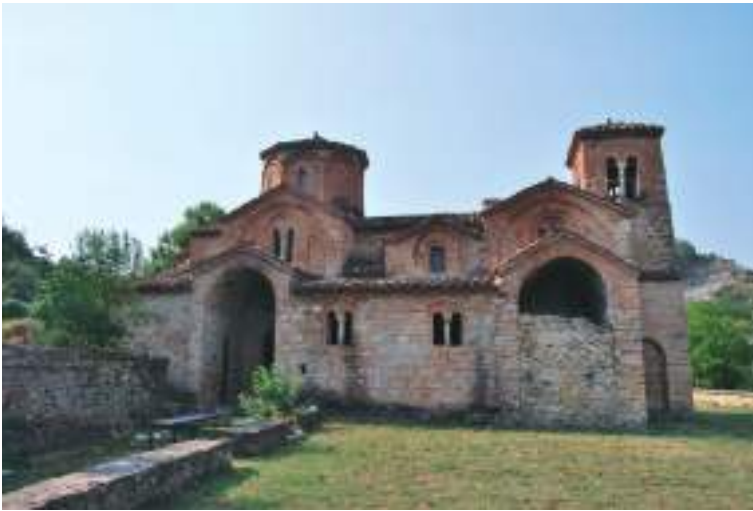
Figure 1 Church of Saint George (North view). 11th-13th cc. Brickwork. Omorfokklisia, Kastoria, Greece. © Elena De Zordi
