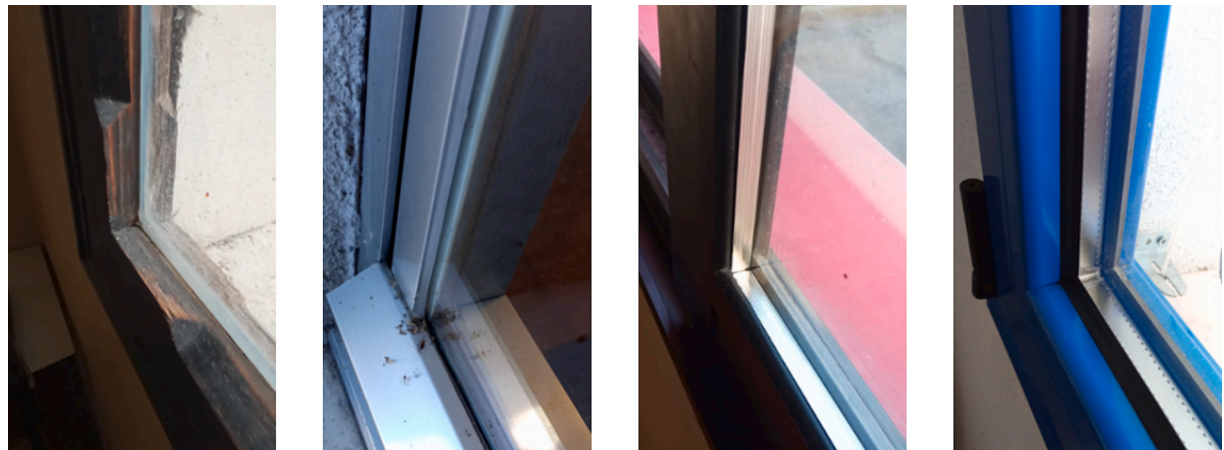
Fig. 6. Windows (from left: single-glazed wood frame, single-glazed aluminium frame, double-glazed aluminium frame, double-glazed PVC frame).
