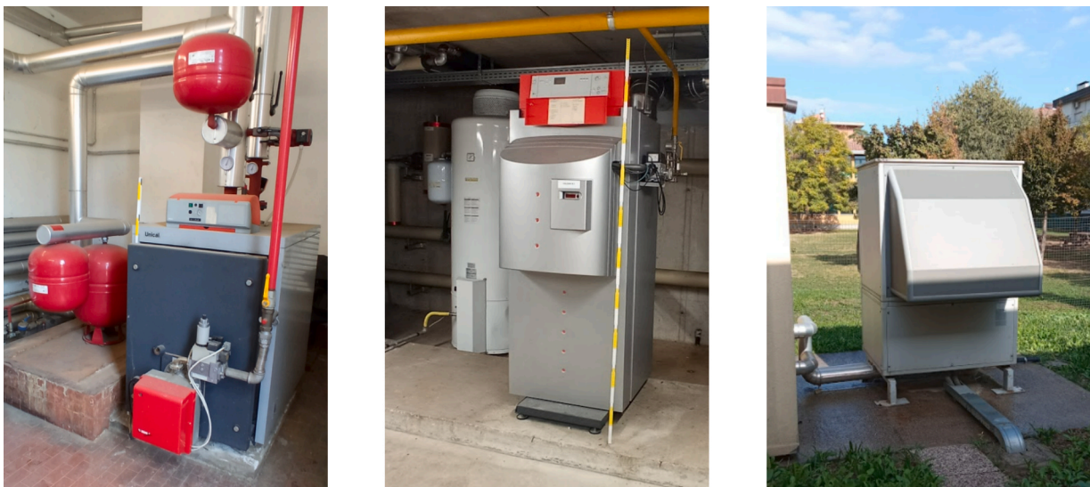
Fig. 4. Heat generators (from left: traditional boiler, condensation boiler and heat pump).
