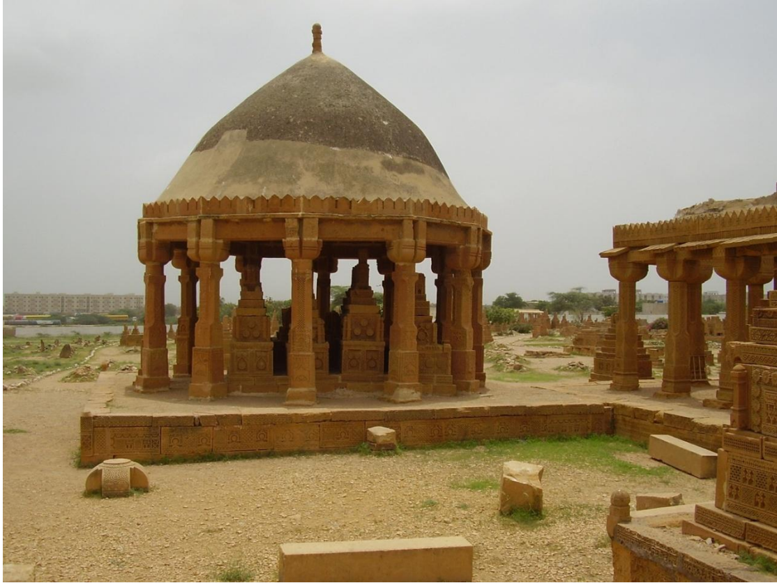
Fig 33(a). Umbrella shaped canopy ( chhatris ) External and internal views constructed over 12 pillars.
