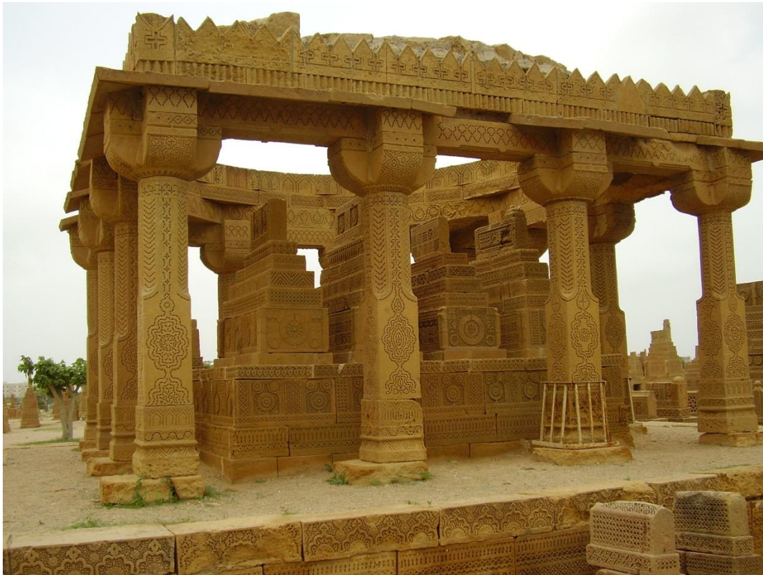
Fig 35 .Close look of the Square shape canopy constructed over 12 columns.
