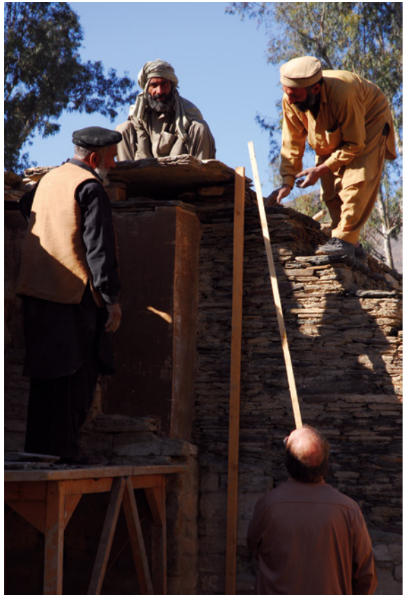
Figures 2-3 Restoration in progress at Saidu Sharif I. 2012 (ACT; photo by Fabio Colombo)
