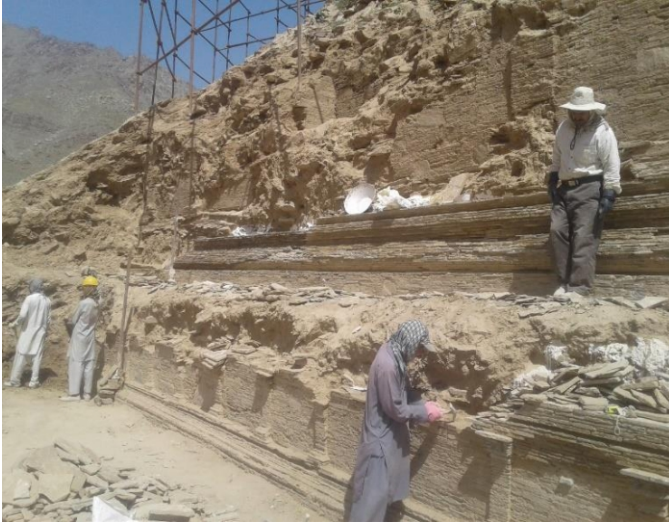
Fig. 25: Excavation of Top Dara stupa
