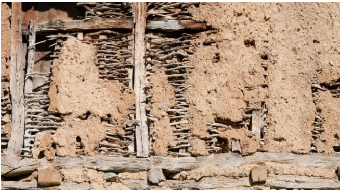
Fig. 47: Wattle and daub construction system in the 19th century Razboishte monastery, Bulgaria.
