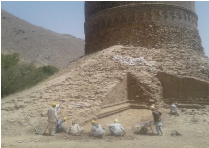
Fig. 4: Excavation at Top Dara stupa
