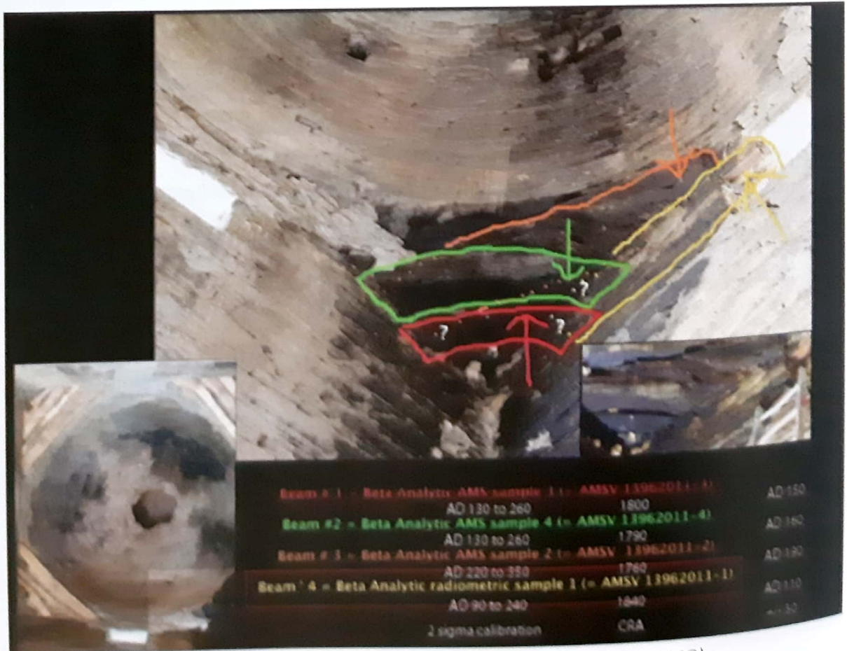
Fig. 64 - The same as above with metadata (Processed by LMO). Note: instead of 'Beam ' 4', read 'Lintel 4'.
