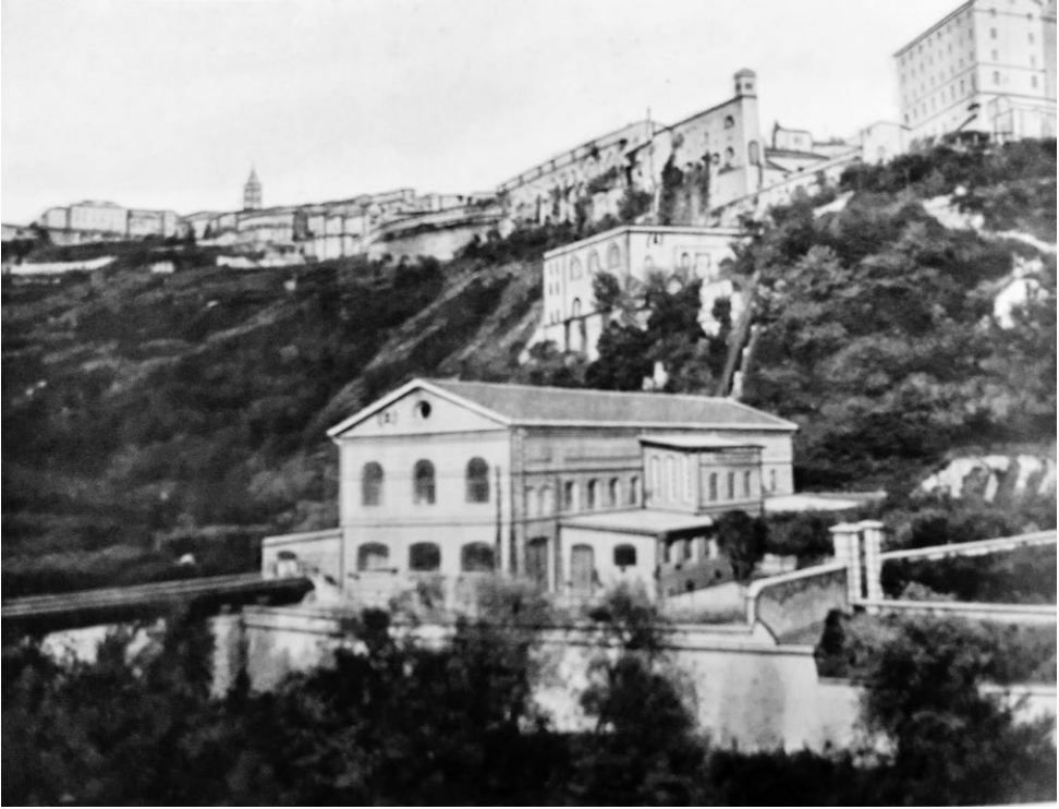
Figure 4: The new power station of Tivoli
