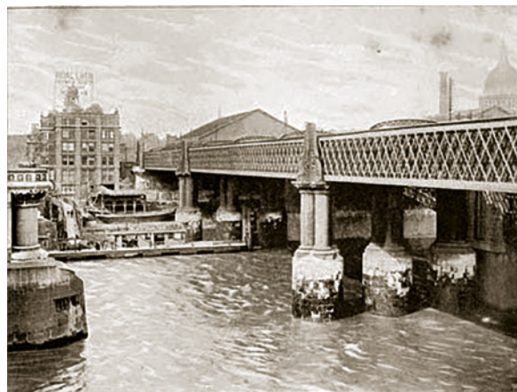
Figure 14 Joseph Dredge, Thames Bridges, from the Tower to the Source , London: Engineering , [1897], Pl. 6 ( Blackfriars Railway Bridge ). © Wikimedia Commons
