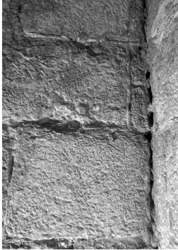
Figure 14.5 Level 2, niche 8: the rubané joints (photograph by C. Tonghini)
