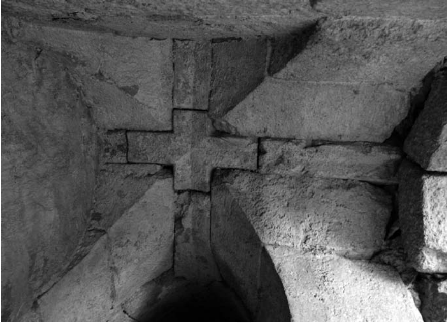
Figure 14.6 The vaulting of the staircase (photograph by C. Tonghini)
