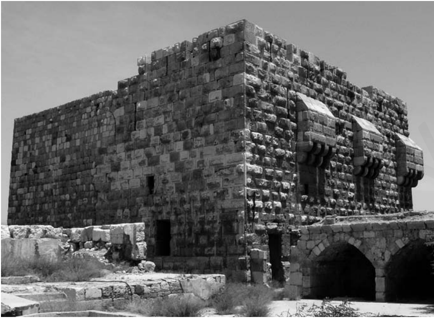
Figure 14.2 Upper part of tower 8, from the south-west; on the west façade the part on the left corresponds to the reconstruction of Period IV (photograph by C. Tonghini)
