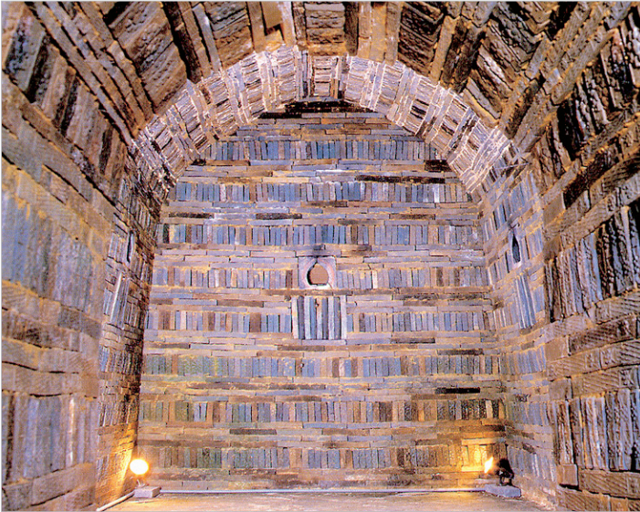
The brick tomb of King Muryeong of Baekje | © Cultural Heritage Administration The tomb of King Muryeong was built with bricks after the Chinese style. It is located in Gongju-si, Chungcheongnam-do.
