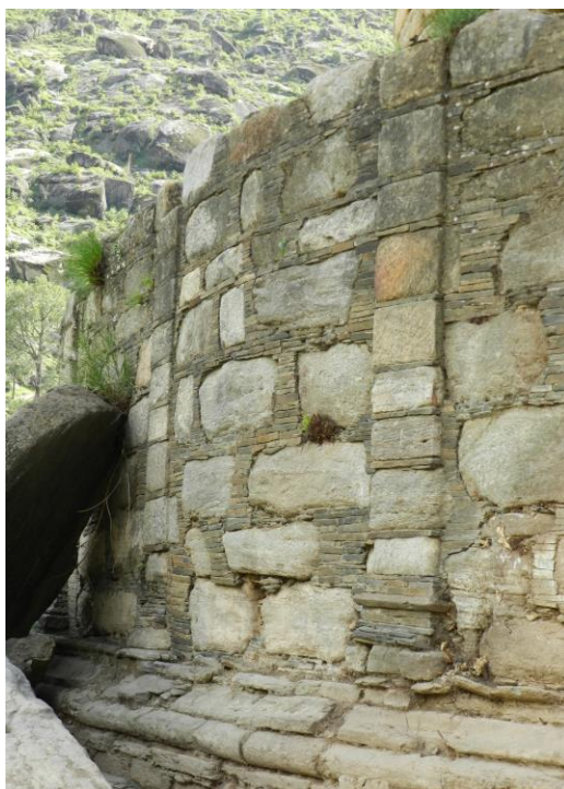
Figs. 22-24 - Restored masonry (2nd storey; 1958-59). (Photo by LMO).
