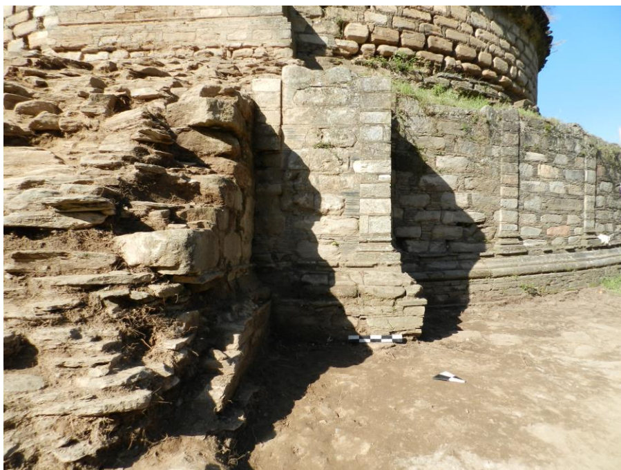
Figs. 48-50- Top of the 1st storey: The 4 floors on the W side (left). The lowest one [14] corresponds to [39] on the E side. (Photos by LMO).
