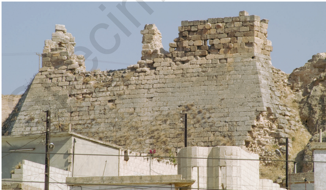
Fig. 5. The glacis from the west, with the crowning parapet. Photo L. Tarducci.
