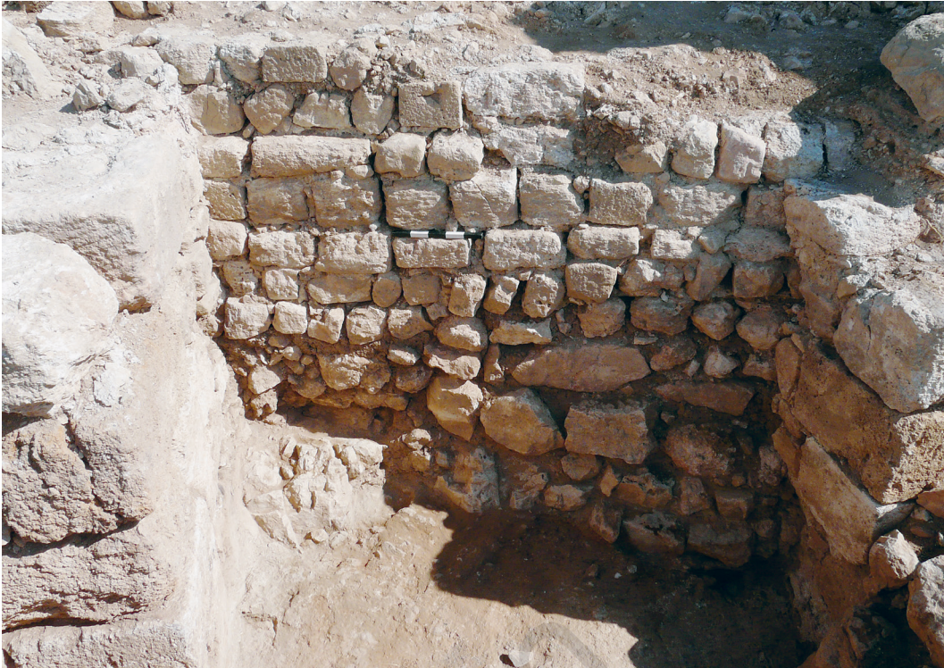
Fig. 8. The inner wall of the newly excavated building (Fig. 7, sondage B), from the west. Photo C. Tonghini.
