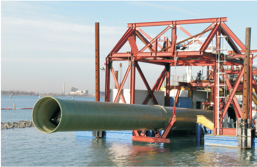
Fig. 1: PIF pipeline laying operations.
