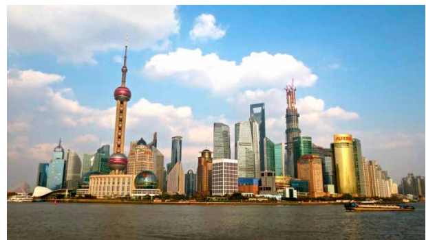
Fig.17. Actual view of Pudong from the Bund
