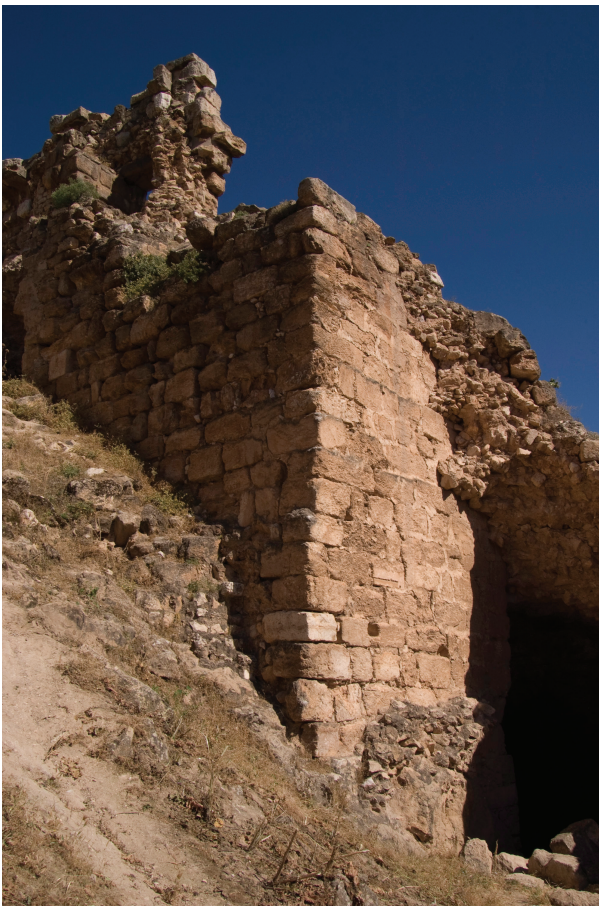
FIG. 3 BUILDING CF6 FROM THE SOUTH-EAST (PERIOD II).
