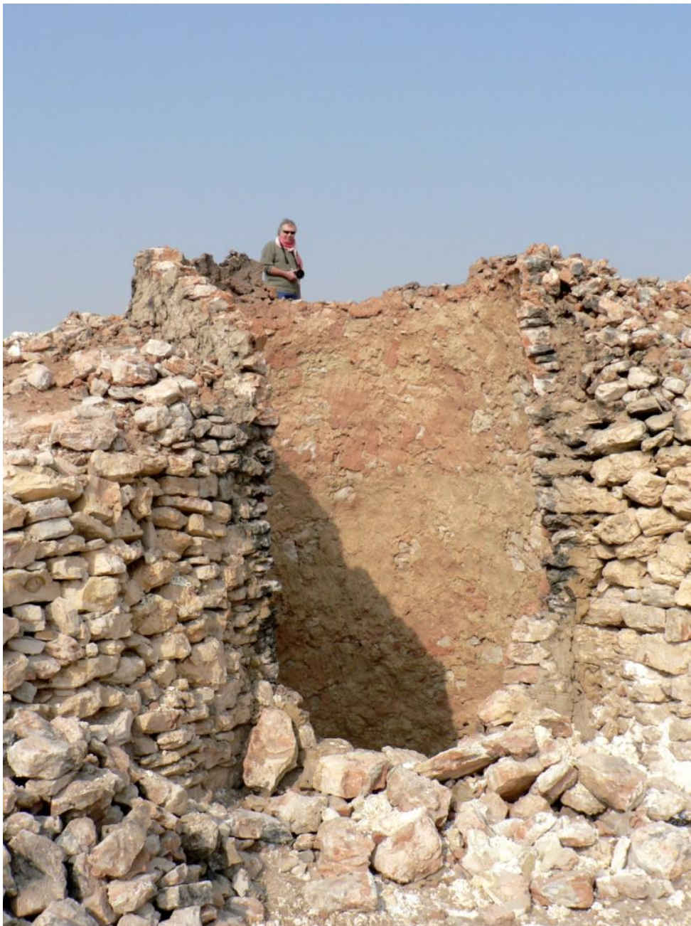
Fig.2: A recently used kiln for lime production, site B ( Author's photograph ).
