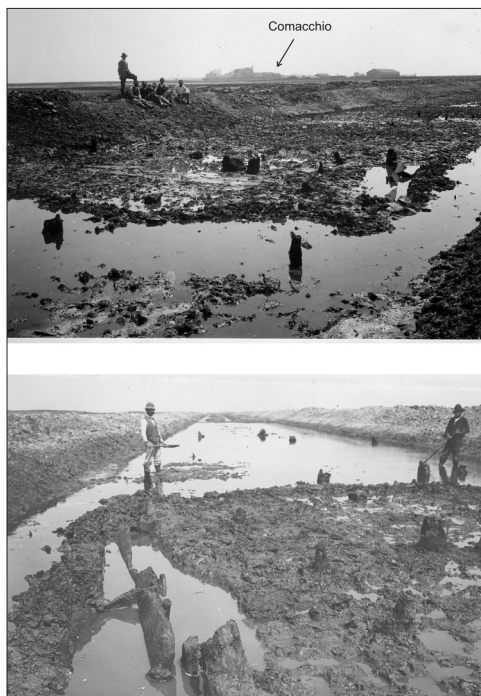
12. Comacchio: Valle Ponti. Photos taken during the excavation works of the drainage channel with the recovery of wooden poles and planking pertinent to the port structures.
