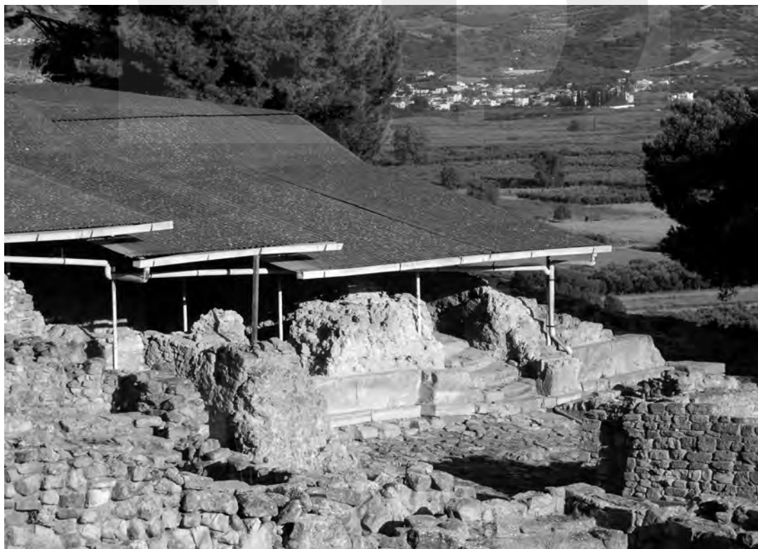
Fig. 2 - The three-floored South-West Building with its orthostat façade on the Lower West Court, from North-West
