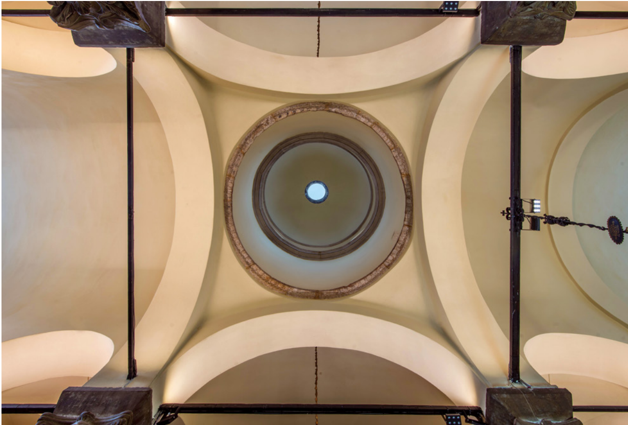
Figure 1 Church of San Giacomo di Rialto, Venice. Network of metal struts supporting columns and arches
