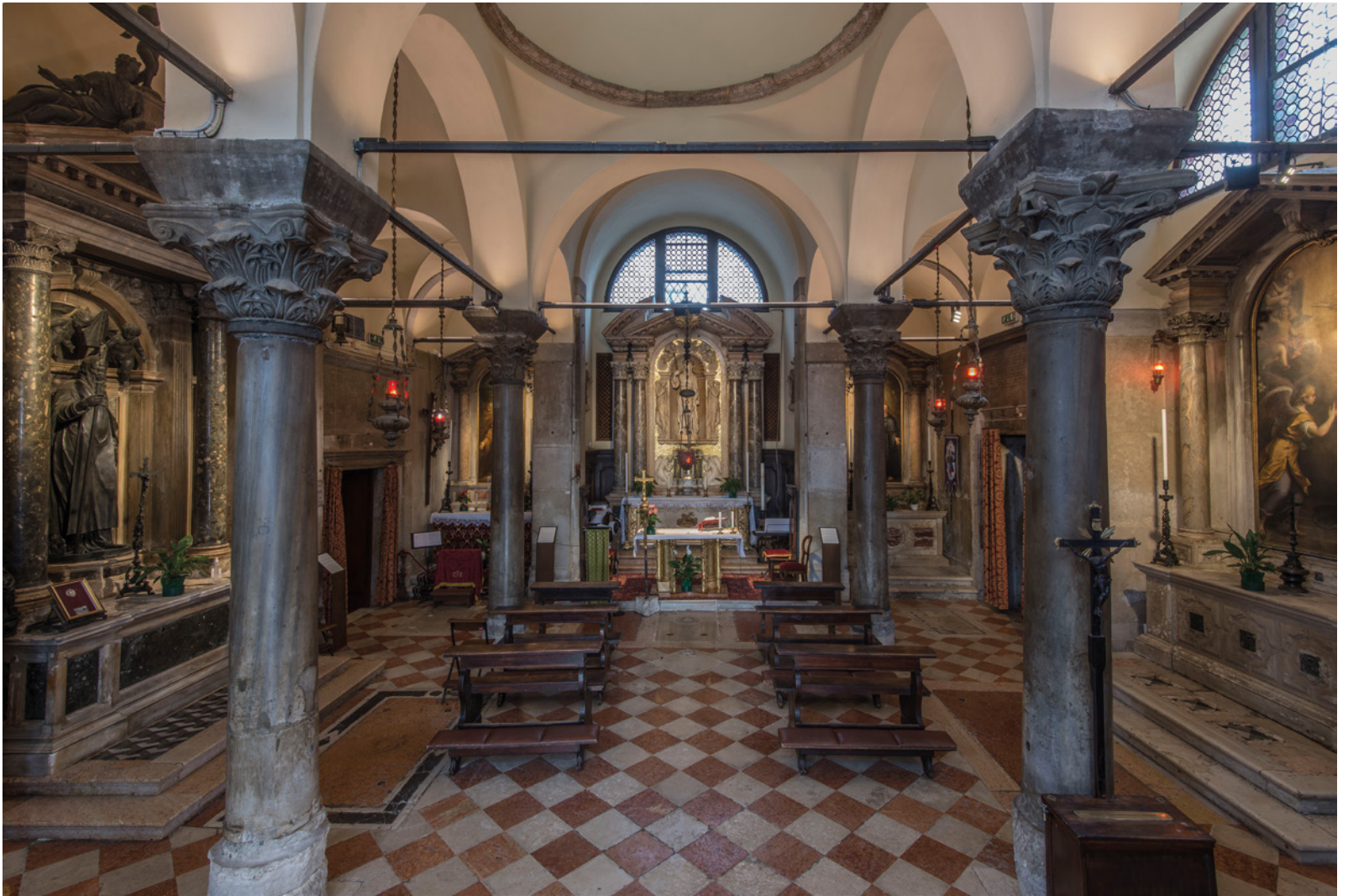
Figure 2 Church of San Giacomo di Rialto, Venice. View of the interior with the main nave with two rows of three columns made of Proconnesian marble. Photo © Böhm
