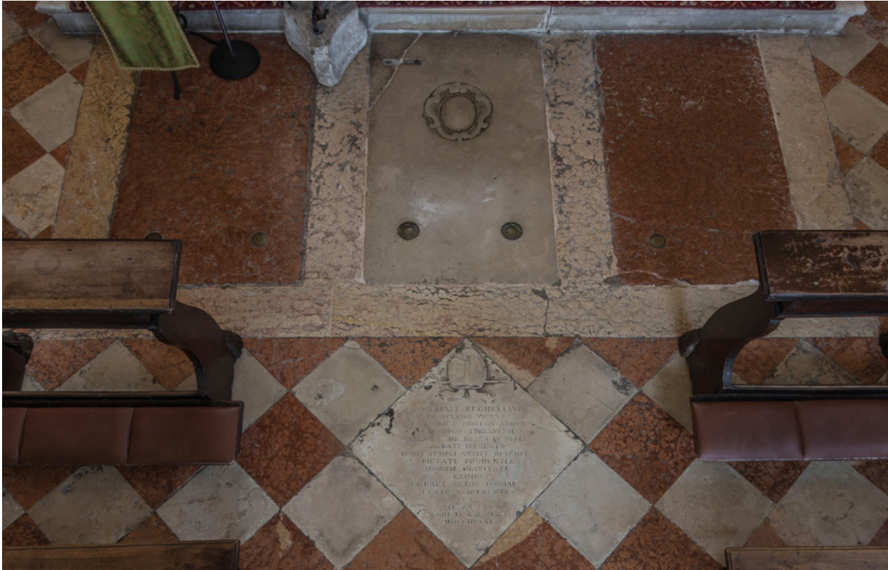
Figure 1 Church of San Giacomo di Rialto, Venice. Pavement with a chequerboard pattern consists of squares of white Istrian stone and red Verona broccade. Photo © Böhm
