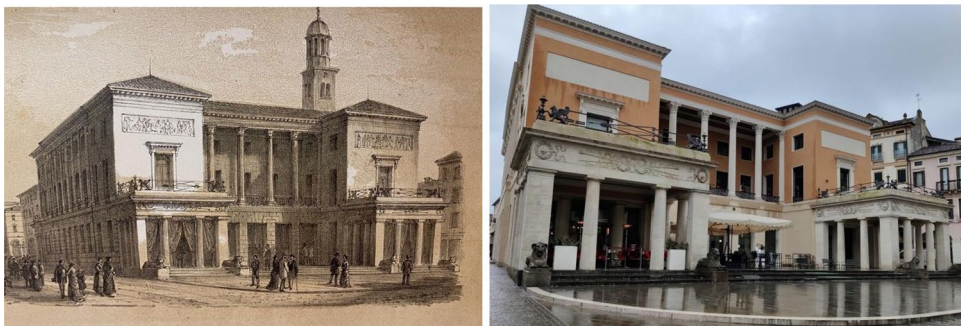
Figure 1. Caffè Pedrocchi at its founding (from Pedrocchi, D.C., 1881) and today (authors' photo).
