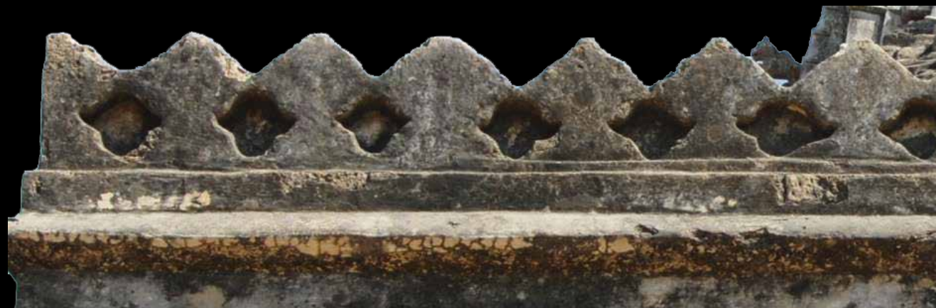
Figure 20. Merlons above the entrance wall
