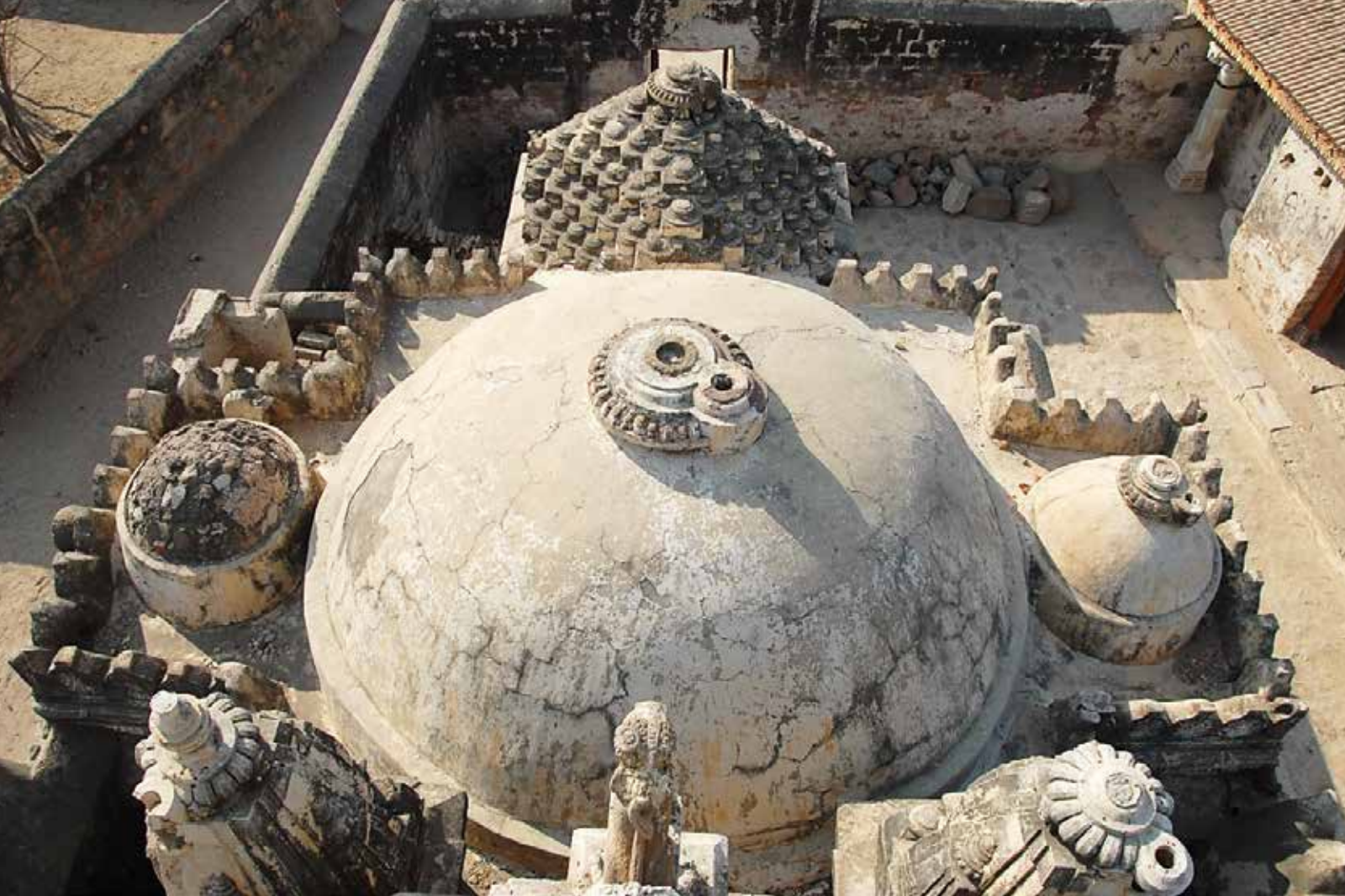
Figure 4. Roof of Mandapa and Ardhamandapa
