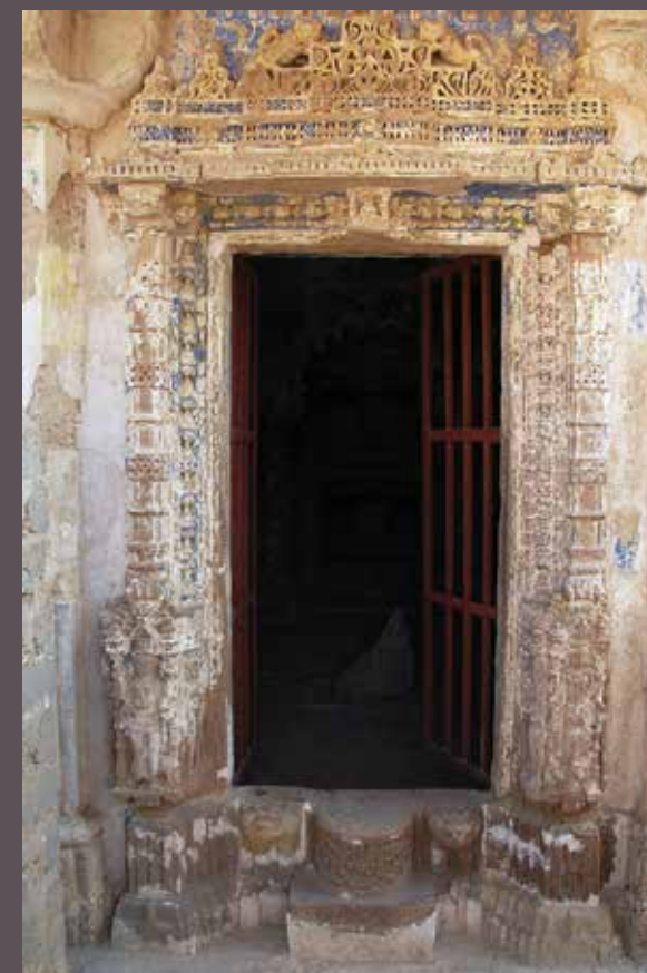
Figure 13. Door Frame of Mandapa
