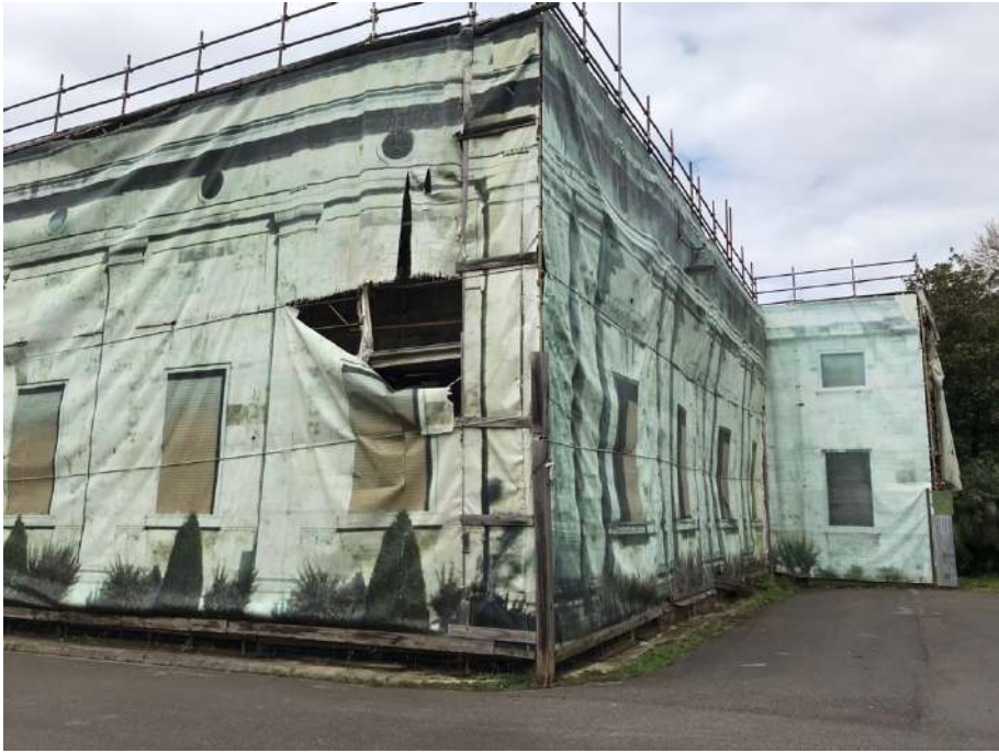
Figure 2. Scaffolding with a torn screen, Montecatini Terme, Italy, 2019. From author's personal collection.
