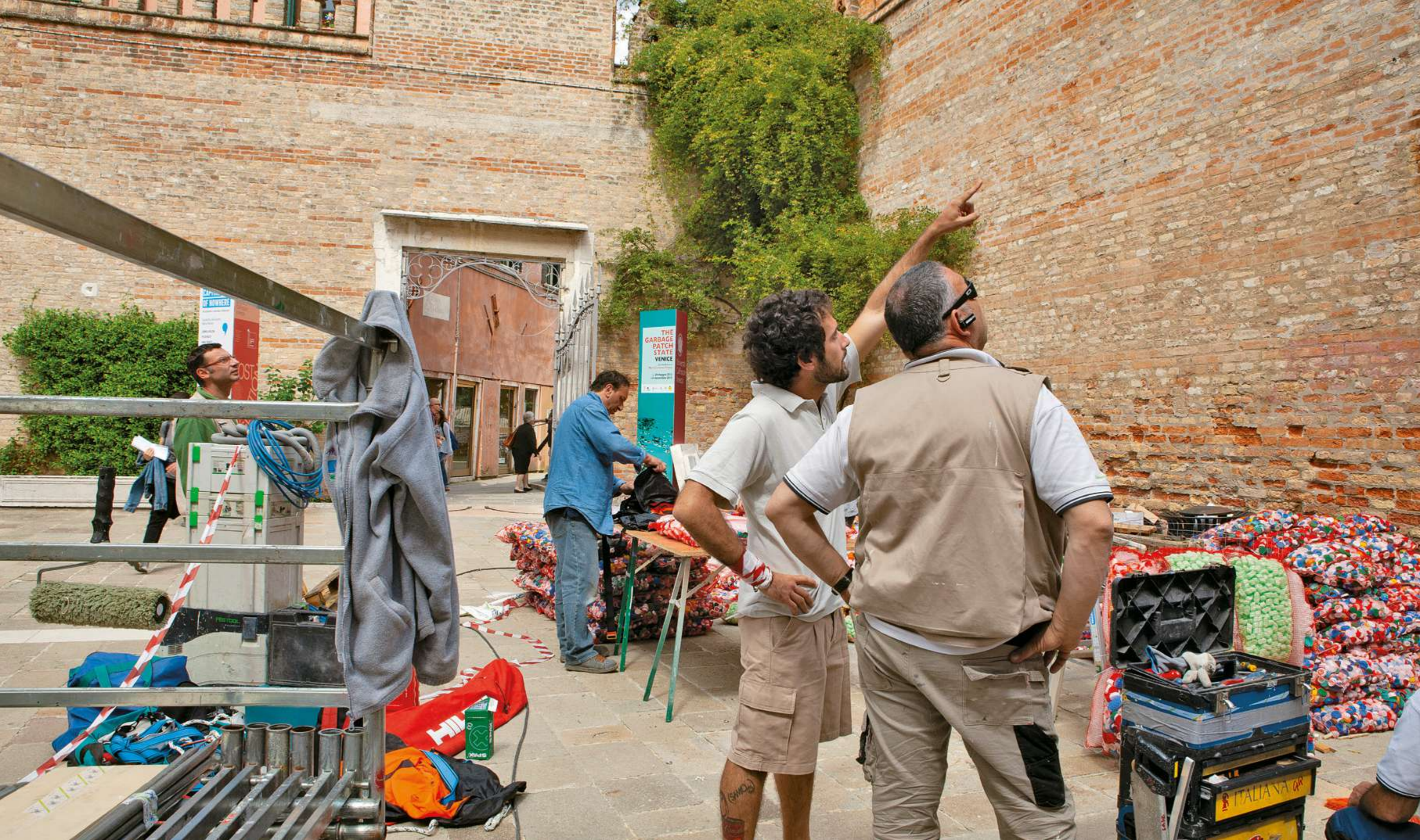
A phase of the installation
