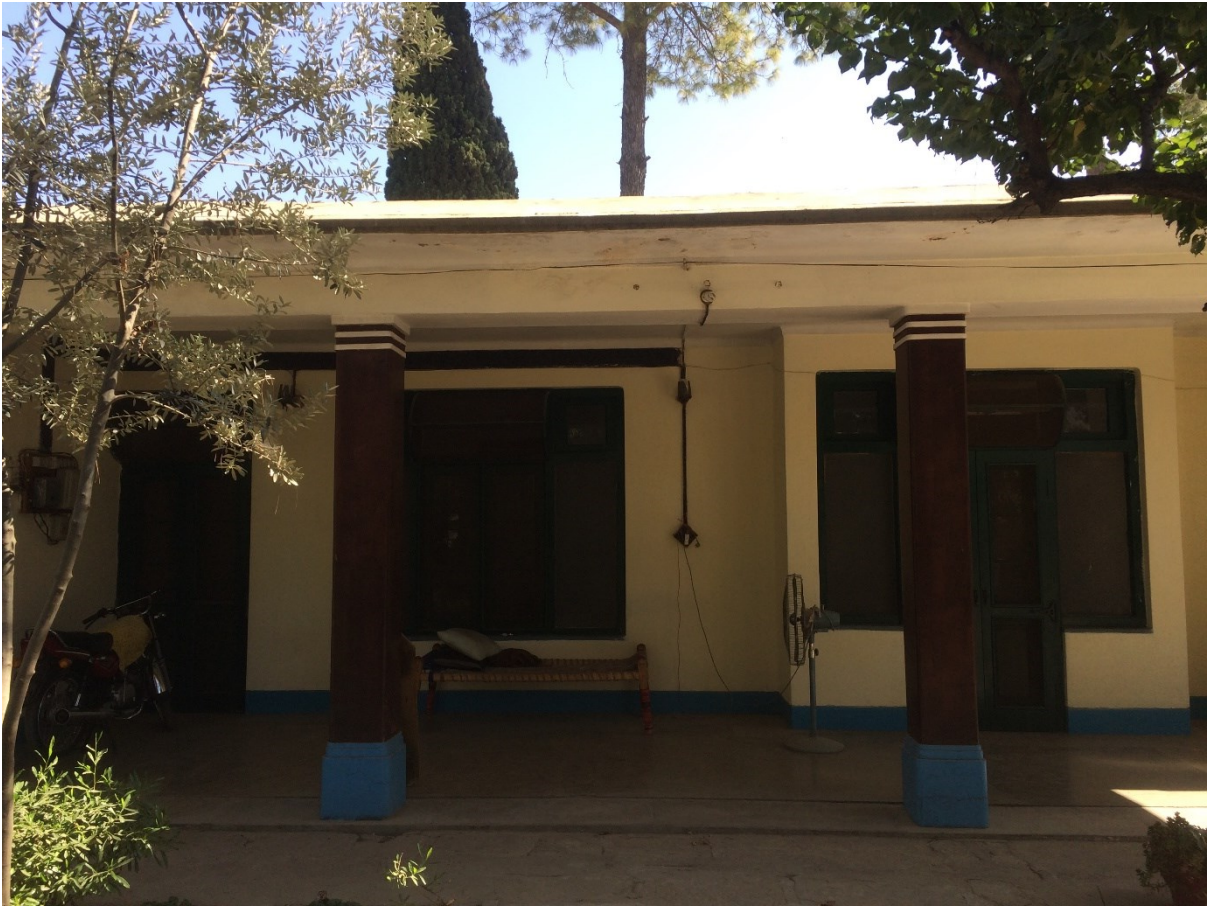
Figure 9. The Mission House: the same verandah of Fig. 8 in 2021.
