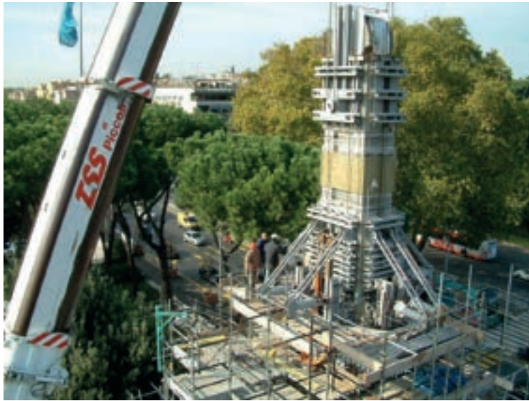
Figure 7. The stele during the disassembly process, Rome, 23 November 2003. Courtesy of Lattanzi Srl www.lattanzi.it
