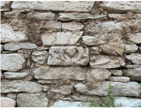
Fig. 15 – Gumbatuna: decorated architectural element reused in the retaining wall of the road leading to the archaeological site
