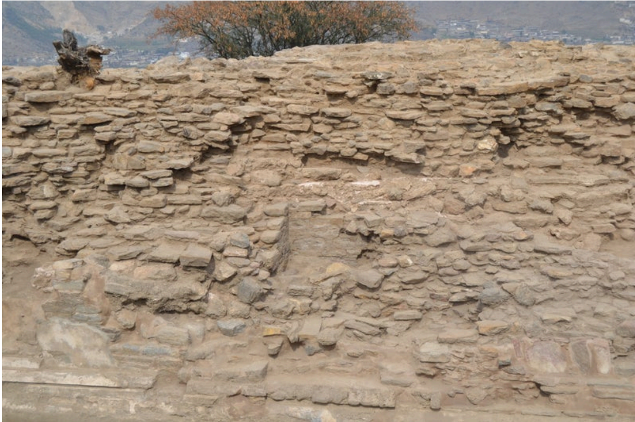
Fig. 50. Temple 6, south side of the podium: evidence of the upper podium floor of the temple of Period 2a (IAMP, CC BY-NC-ND 4.0)
