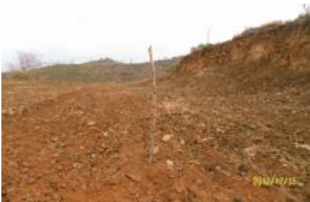
Fig. 15 - General view of WGB (s-IV) after bulldozing.
