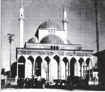
The Shkodër mosque (Hamdi Bushati, Shkodra dhe motet, v. 1, Rozafat, 1998, 125)
