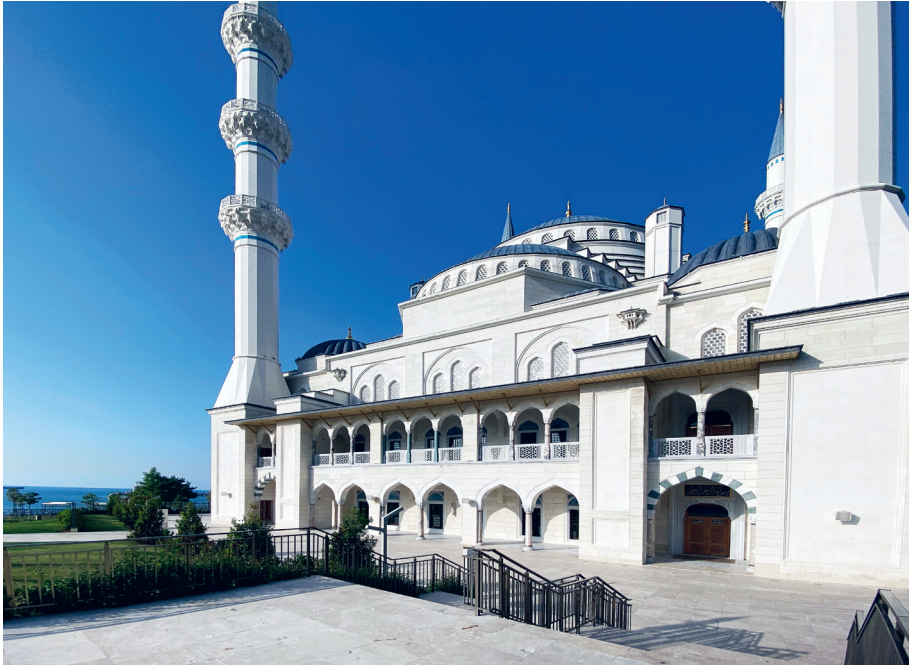
Zonguldak mosque. Photo by the author, 2023
