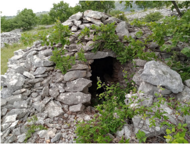
Figure 3: A dry stones shelter ("capanna") built by a farmer from the "spietramenti" stones, as it appear nowadays. [Courtesy of Angiolina De Angelis]
