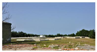
Fig. 9 Nardello US Air Force radar station. Square concrete platforms served as bases for radar dishes
