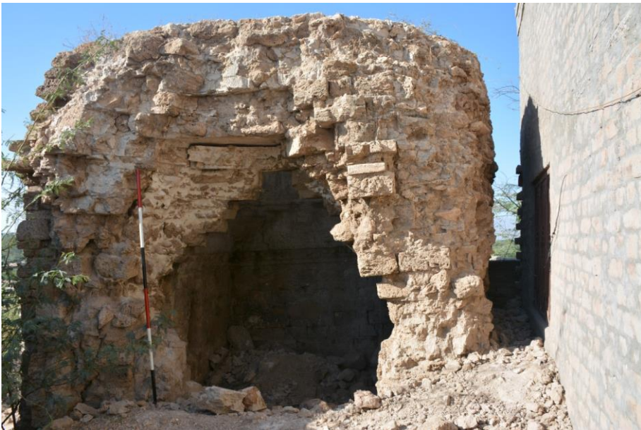
Fig. 6 – A view from the east, condition eight months before destruction (HKL).
