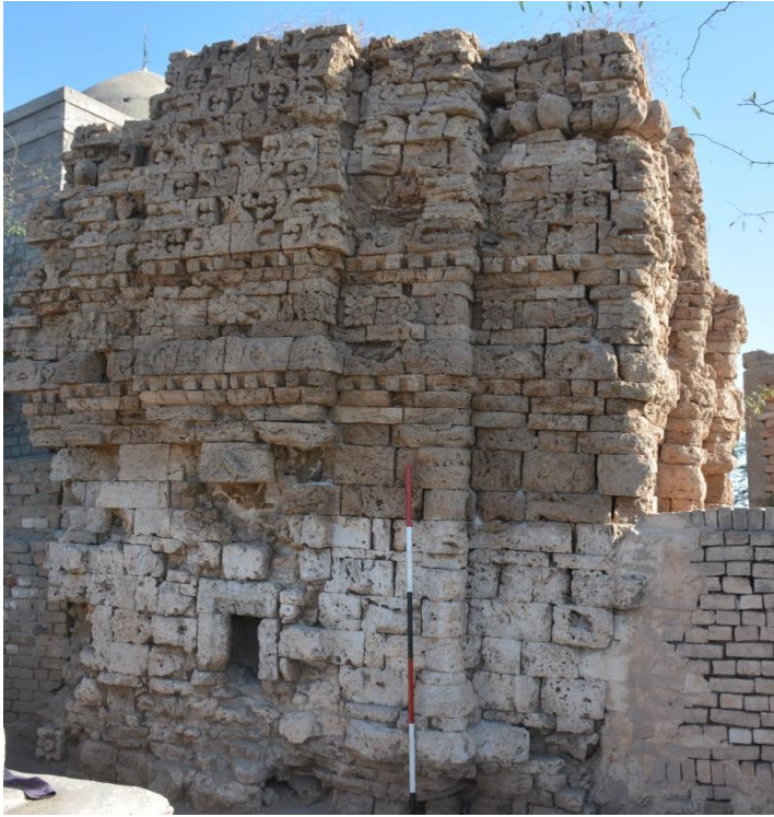
Fig. 3 – Temple from south-western side (HKL).
