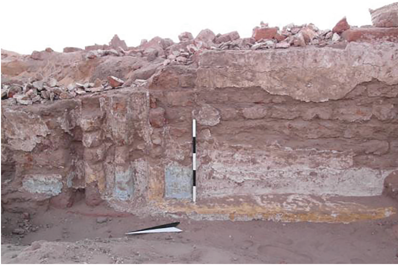
Figure 10. Section of the western façade of Palace B1500 with polychromy (photo by M. Gottardo).
