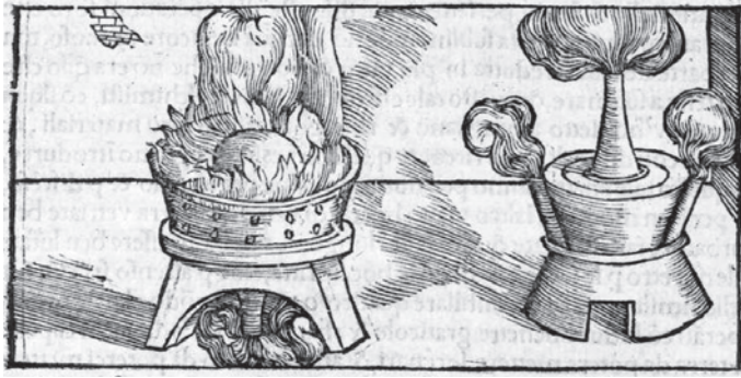
Fig. 3. De la Pirotechnia (Book IX, 130, verso). Sublimation devices (courtesy of The History of Science Collections, University of Oklahoma Libraries).
