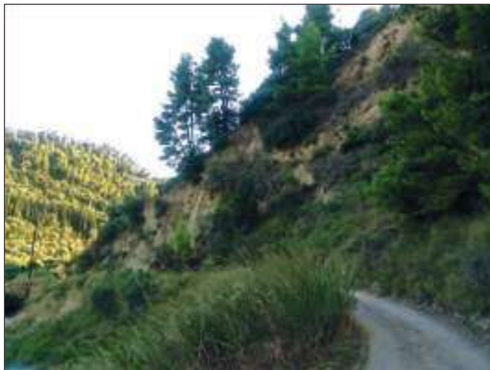
b) The modern road leading to the site from northeast (Photograph: A. Mercogliano)
