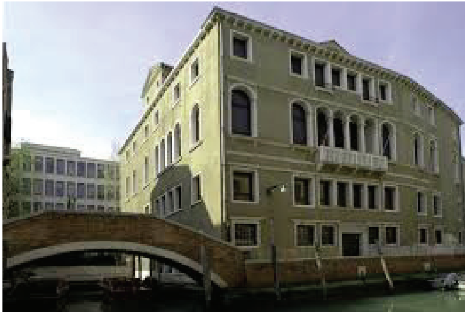
Figure 3.2 Malcanton Marcorà Palace, Library of Humanities, Ca' Foscari University of Venice (Italy).
