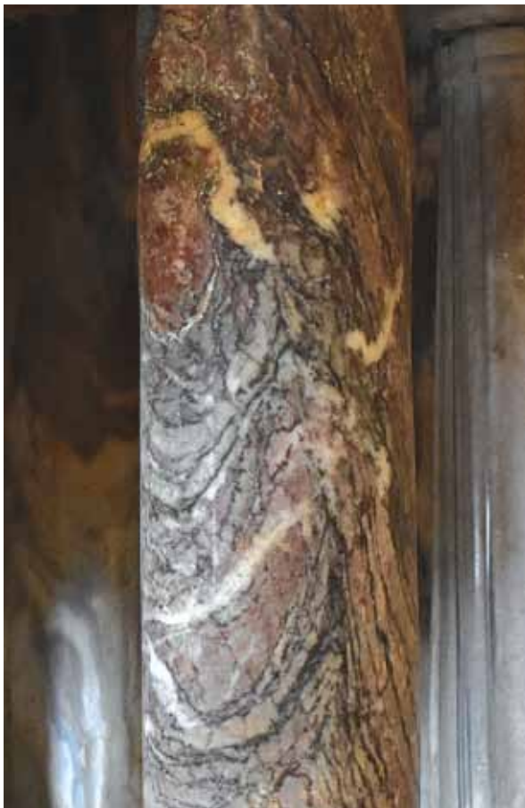
Fig. 6 - Detail of Fig. 5 showing the wawing schistosity of the cipollino with red and green bent layers.
