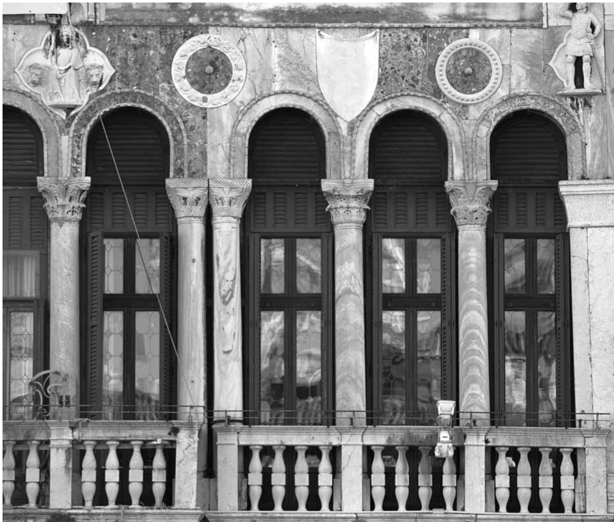
Fig. 7 - Detail of the polyphora of the piano nobile of Ca' Loredan with columns, capitals and reused slabs.
