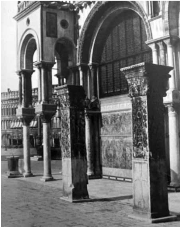
Fig. 10 - The 16 th -century plugging of the Porta da Mar of the Basilica of St. Mark, featuring a marble facing added after 1504. The facing comprises deteriorated Proconnesian marble slabs arranged in the macchia aperta (book-matching) technique. The photograph predates the 1880 marble replacements.
