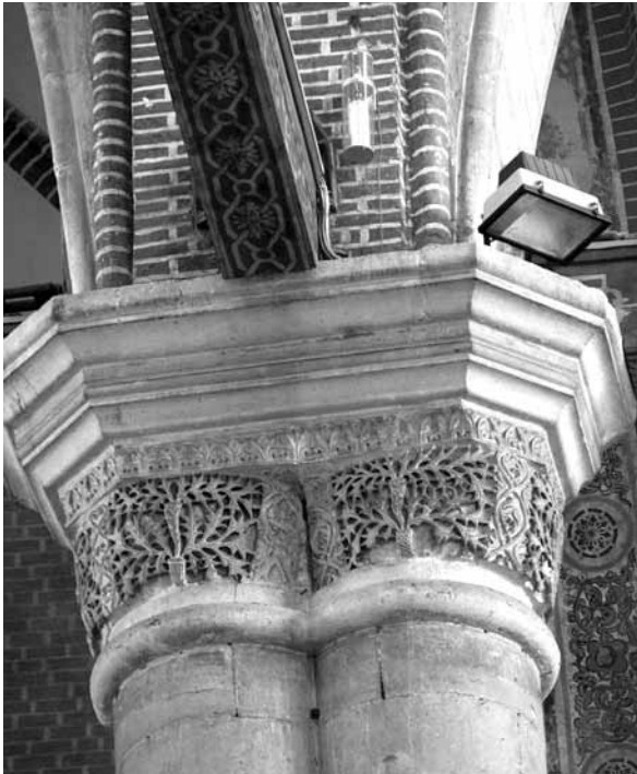
Fig. 3 - Venice, Basilica of Sts. Giovanni e Paolo, main nave, polystyle pillar with Byzantine capitals.
