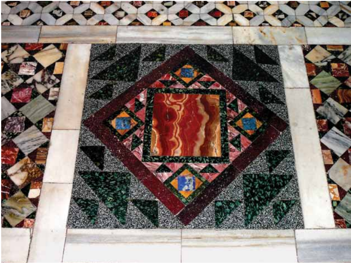
Fig. 15 - Left side of the altar of the Nicopeia , square of alabastro di Castelnuovo dell'Abate inscribed in a larger one filled with triangles of serpentino and granito verde fiorito di bigio .
