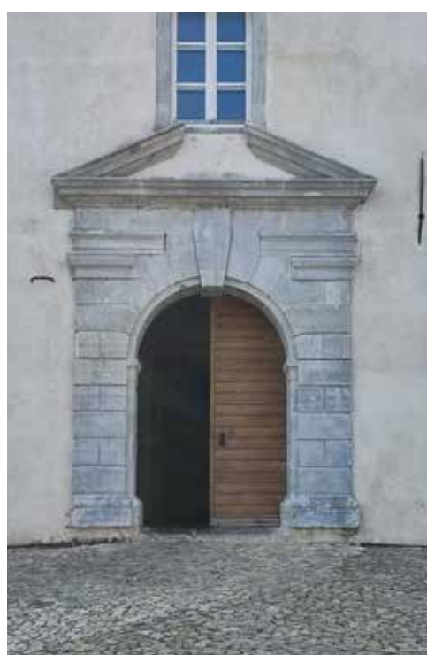
Ill. 3.27. Zrinski Palace, Nova Kraljevica, external gate, completed in 1653
