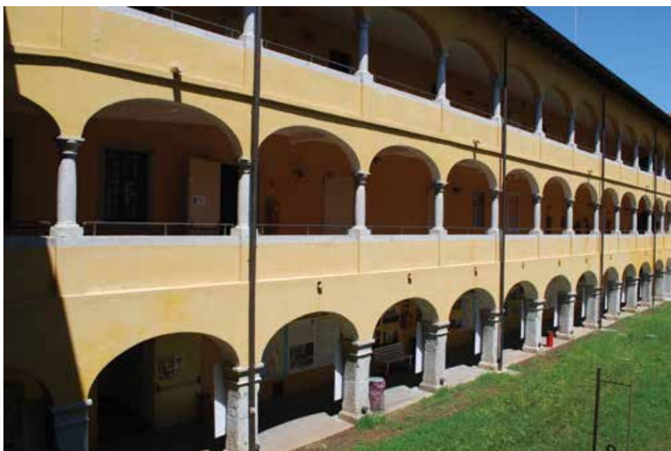
Ill. 3.45. Wendenberg Palace, Gorizia, courtyard, 1634–1649
