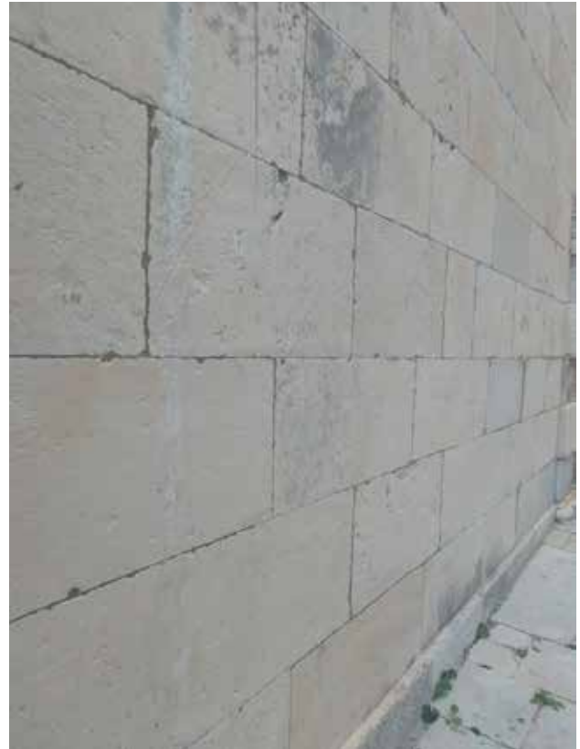
Ill. 3.1. Church of Our Lady of the Rosary, Dubrovnik, engraved proportional system, east façade, begun in 1594 (Guarneri)
