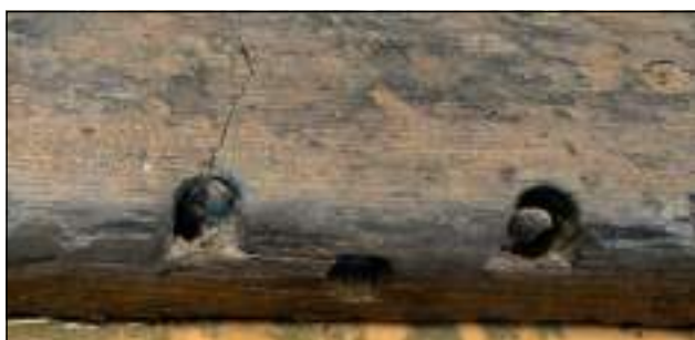
Fig. 14.19. Wooden dowel along the edge of the plank of Roman period found on the shore at Grado (photo: E. Costa) (authorised by the Soprintendenza ABAP FVG-MIC, duplication forbidden art. 108, co.3 del D. Lgs 42/2004 s.m.i.).
