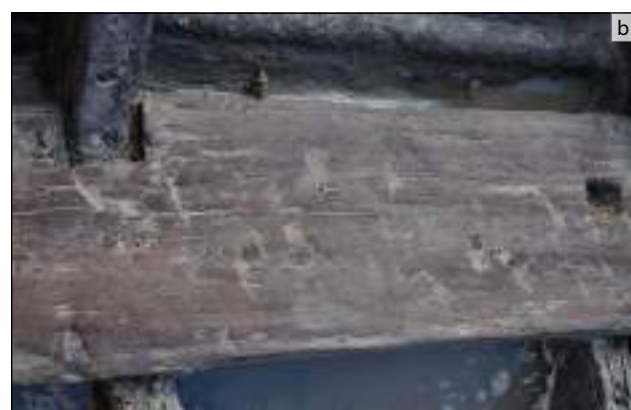
Fig. 9.23a-b. The ceiling plank connected to frame F9 with an iron nail (photo: E. Costa).
