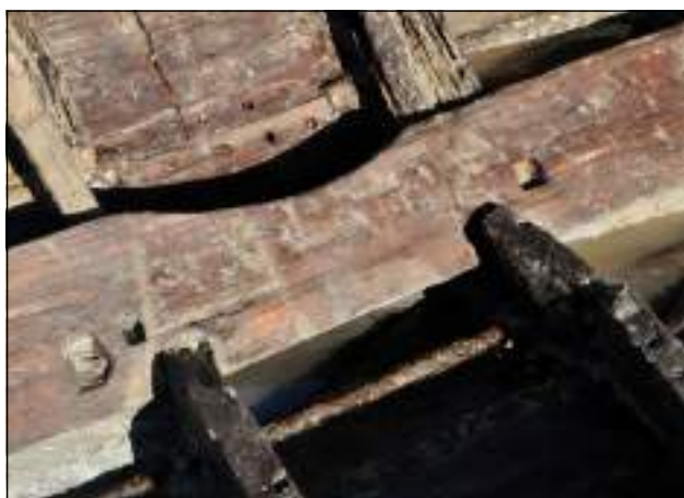
Fig. 9.25. The quadrangular recesses and the curvature of the ceiling plank in the central area, between the frames F12 and F13 (photo: E. Costa).
