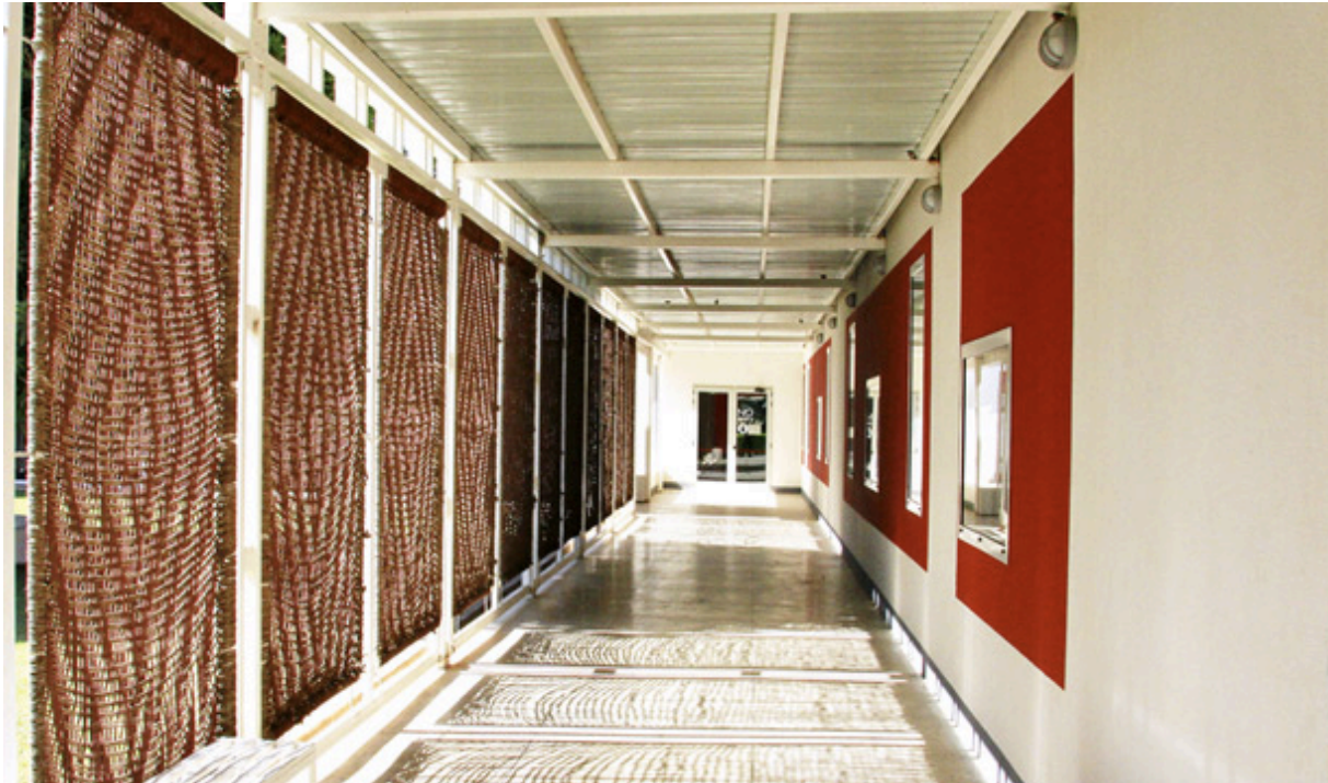
Fig. 2: A detail of the porticos of the Salam Centre with the twined vegetal panels on the left and the small double-screen windows on the right (photo by Emergency NGO 6 )
