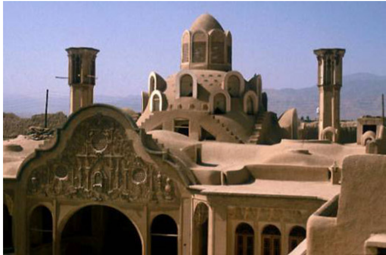
Fig. 3: Two tall wind towers cool the courtyard of Persian Borujerdi ha House (1857) in Central Iran
