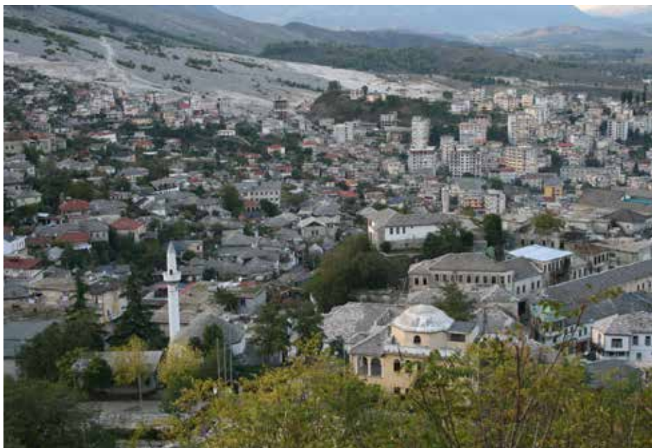
Figure 6. General View of Ergirikasri from the Citadel
